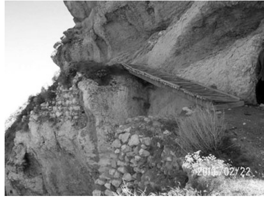
Fig. 6 View of the modern wooden bridge and the original wall foundation of the access road to the fortress
