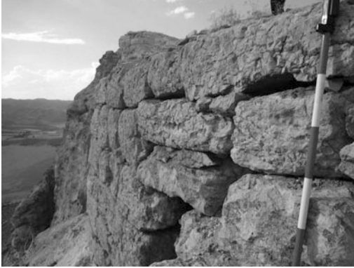
Fig. 13 Detail of the masonry of a wall
