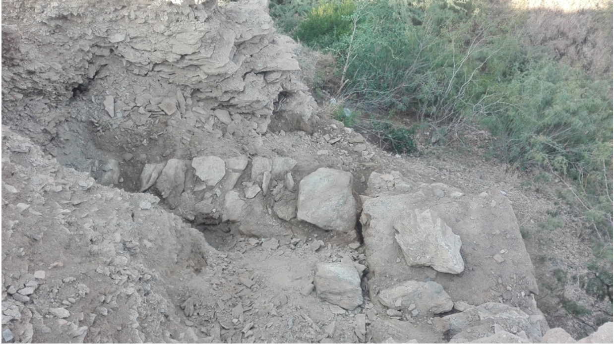
Figure 10. Rubble masonry wall at the north-western corner of Block B1. Due to the threat of potential collapse of the entire retaining wall on the north and west of the corner, it was not possible to go deep to expose clearly the whole wall for proper photography. (Photo: author.)
