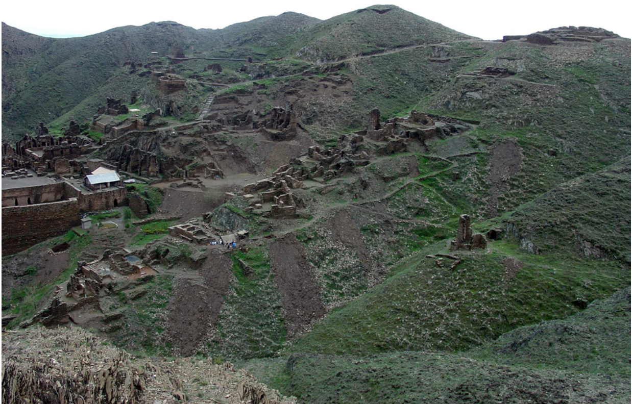
Figure 9. The buildings on the right from top down have been named Block B for the present conservation activities under the US-Funded Project titled ‘To support the Preservation and Conservation of Buddhist Ruins of Takht-i-Bāhī’. The first block from the bottom has been named B-1, where the roughly built rubble masonry wall was exposed during investigation for the reconstruction of the retaining wall on the north-western corner of the block. (Photo: author.)
