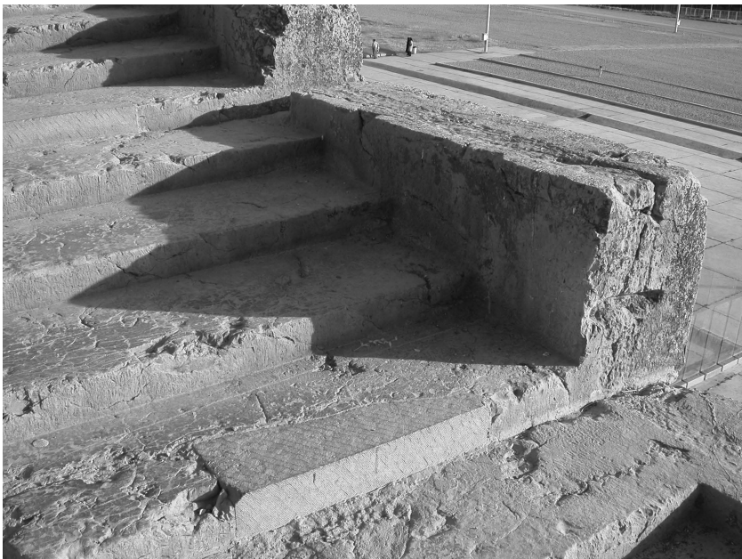
FIGURE 2.6 Persepolis, Grand Stairway, showing several steps and parapet carved in a single stone block (2004)
