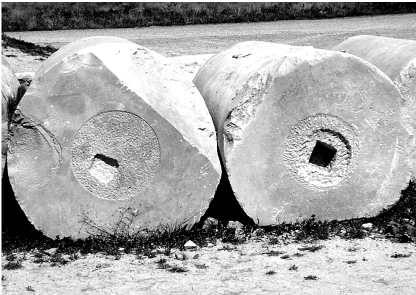
FIGURE 2.4 Pasargadae, column shafts, showing anathyrosis stone carving technique for precision in the joints (1998)
