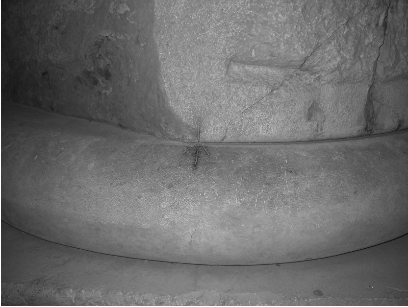
FIGURE 2.48 Signs for matching stone torus and shaft (2006)
