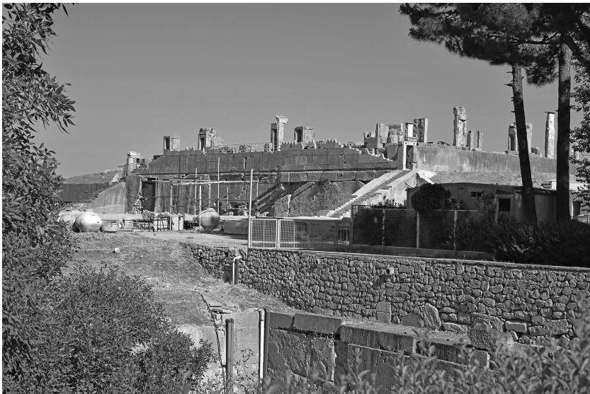
FIGURE 2.35 Palace of Xerxes, southeast view, showing the two lateral stairs of the southern balcony descending to the Harem area (2016)
